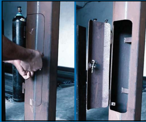
Mid Barrel Hinge c/w Single Locking System
