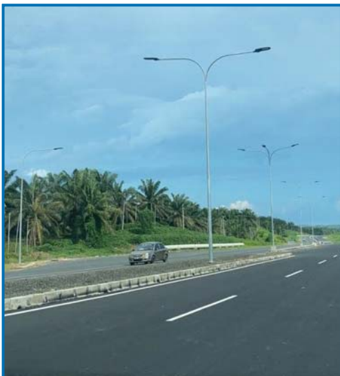
Octagonal Pole WP27 - Pan Borneo Highway, Sabah
