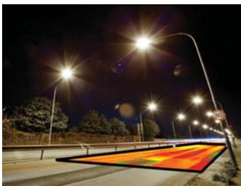
Evaluation of roadway lighting conforming to standards
