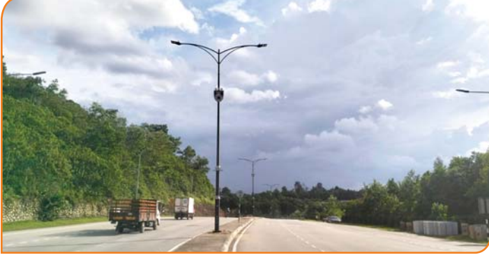
OLE Dura ST at Gelang Patah, Johor, Malaysia
