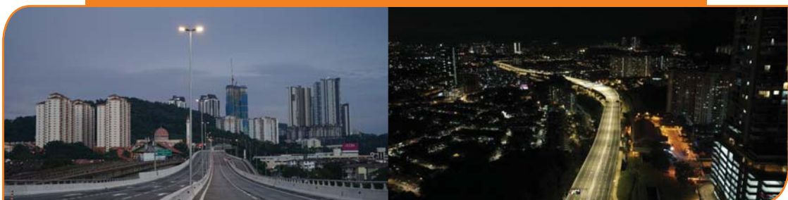
OLE Dura ST at DUKE 3 Highway, Kuala Lumpur, Malaysia
