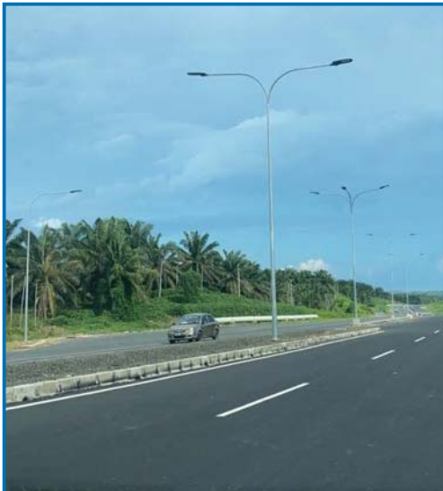
Octagonal Pole WP27 - Pan Borneo Highway, Sabah
