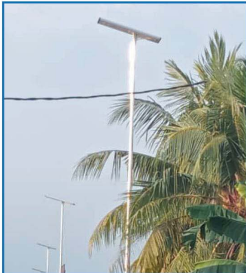
Solar Octagonal Pole Jalan Parit Raja Darat, Johor
