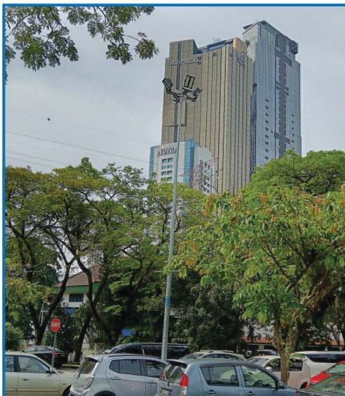
Floodlight Octagonal Pole Parking Padang Astaka, Selangor
