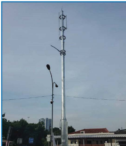
Smart Pole | Monopole Taman Kepong, Kuala Lumpur
