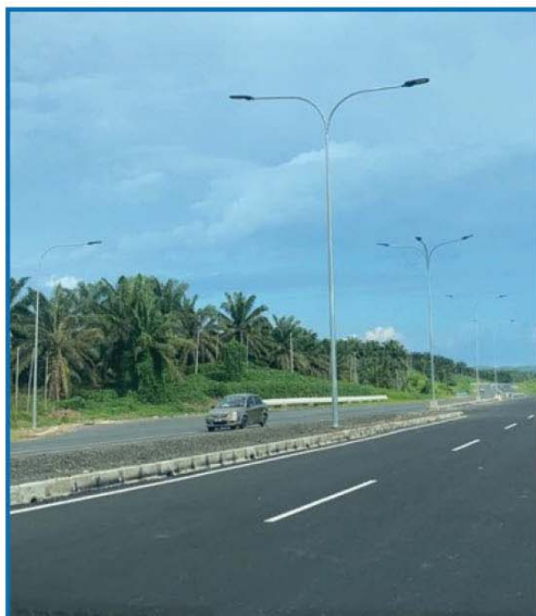
Octagonal Pole WP27 - Pan Borneo Highway, Sabah
