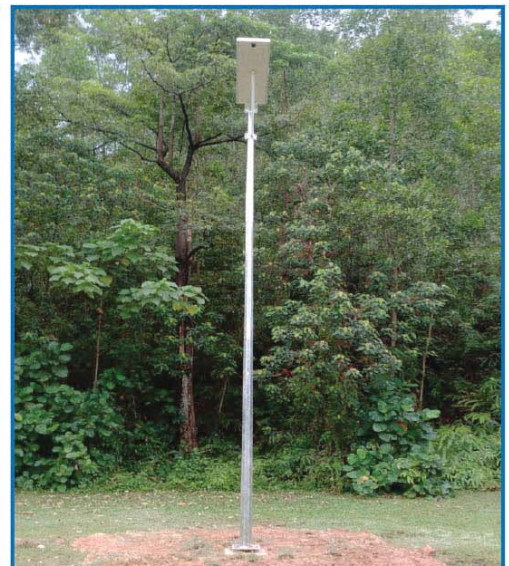
Solar Octagonal Pole Cheras, Selangor
